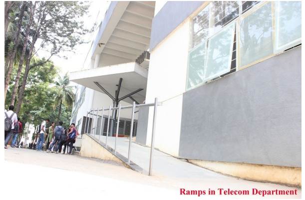
Ramps in Telecom Department
