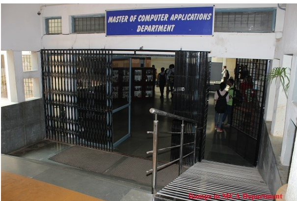
Ramps in MCA Department
